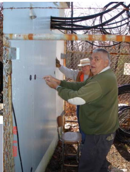
Above: Jim, KC2OGK, fastens insulating panels to the walls of the repeater shack. Left: Tom, N2NZD, installing insulating panels. The inside walls are also insulated to help keep out freezing temperatures.
