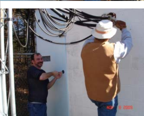
Above: Jim, KC2OGK, fastens insulating panels to the walls of the repeater shack. Left: Tom, N2NZD, installing insulating panels. The inside walls are also insulated to help keep out freezing temperatures.
